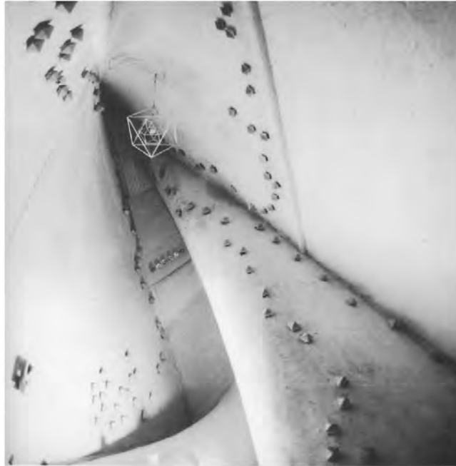
Figure 8.1. View, looking upward, of the inside of the Philips Pavilion. The objects on the surfaces are high-frequency loudspeakers in clusters, the patterns designed by Xenakis. Low-frequency loudspeakers were installed on the ground. (From Treib 1996.)
